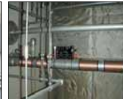
Used for the cooling towers C
